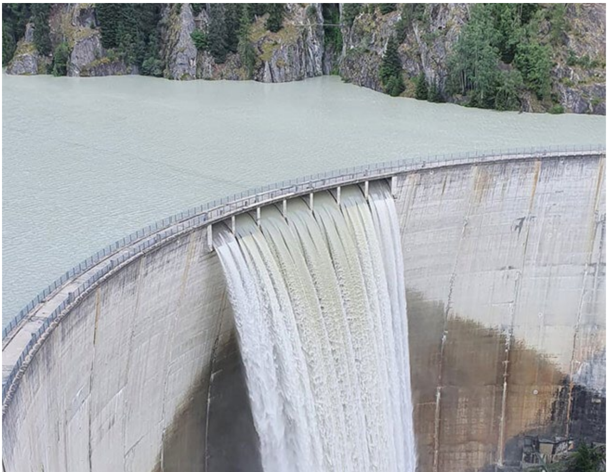
Picture: Gebidem dam. The melting Aletsch glacier brings more water than the power station can turbine. The surplus is diverted over the dam into the Massa Gorge.
