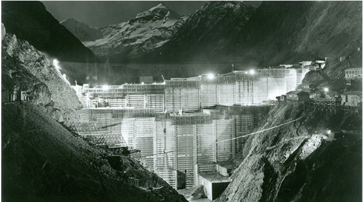
Picture: Construction of the Grande Dixence dam by night – The construction of the dam lasted from 1951 to 1965. Source: Grande Dixence SA
